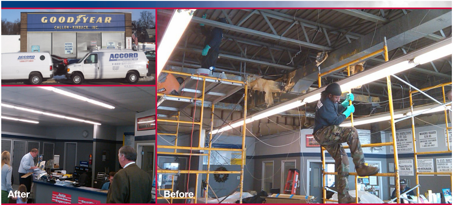
Left Photos: Goodyear of Lemoyne, PA exterior and interior after restoration.
