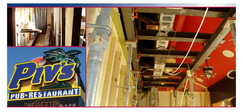
**Left Photo (Top):** The damaged area of Piv's Restaurant had to be supported by steel beams in order for the restoration work to begin.
