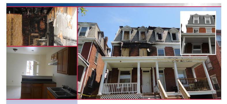
Left Photos (Top): Extensive damage to kitchen area in lower apartment. (Bottom): After gutting the entire kitchen, walls, flooring, cabinets, appliances and countertops were replaced.
